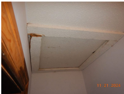
Sealed Access Opening
