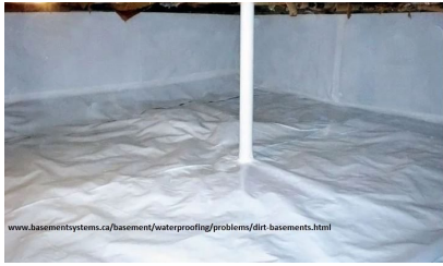
Basement Encapsulation
